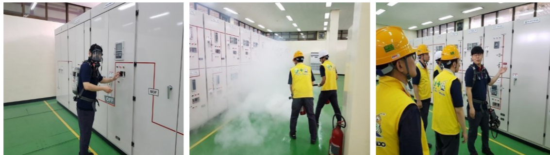
Fire drill for ESS 2) located at the Iksan site
