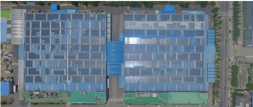
3,000kW photovoltaic generation facility at Iksan site
